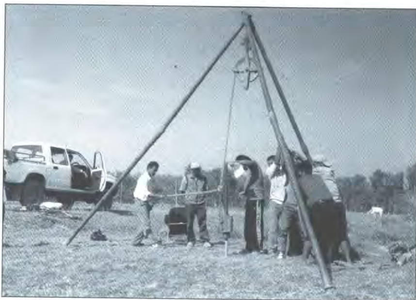
Fig. 3: Performing Standard Penetration Test (SPT) in the field.
