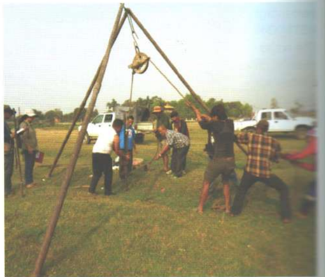
Figure 3: Tripod and site preparation for SPT test
