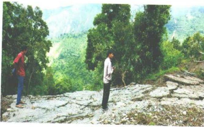
Figure 12: Cracks developed in ground at Ripdada.
