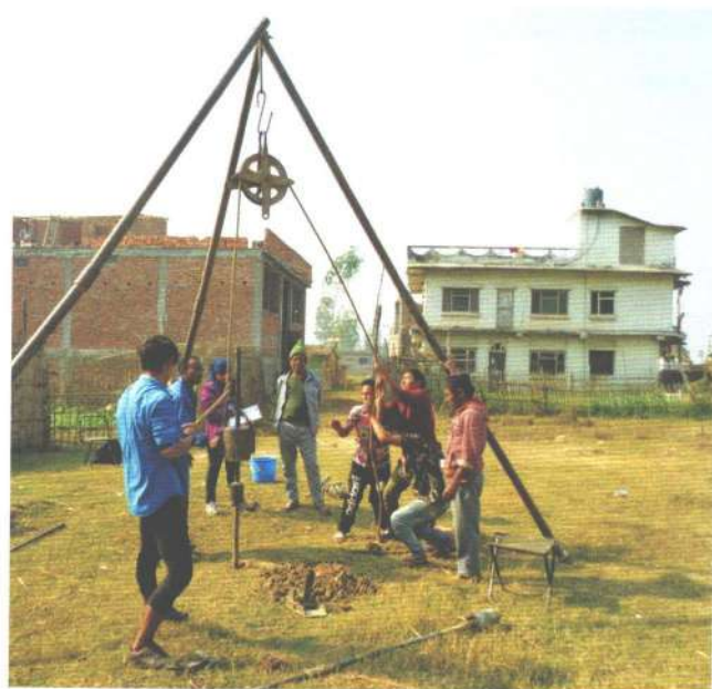
Figure 2: SPT in the field.
