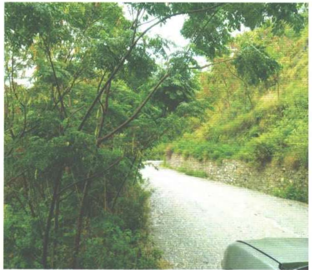
Photo 2: Plantation along access road of Kanchan Quarries
