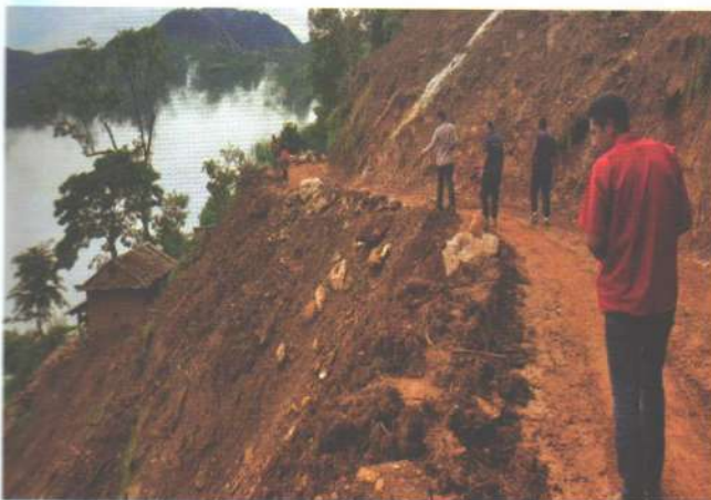
Figure 8: Plane failure of Singdi.
