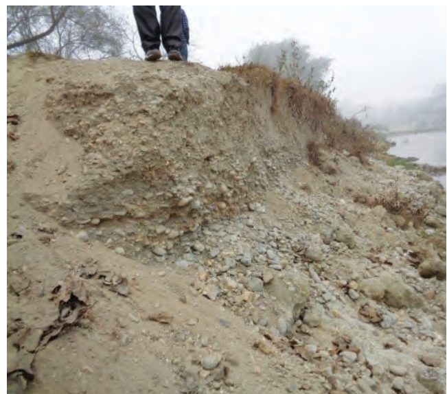
Photo 5: Loose gravel at the bank of Devaniya Khola
