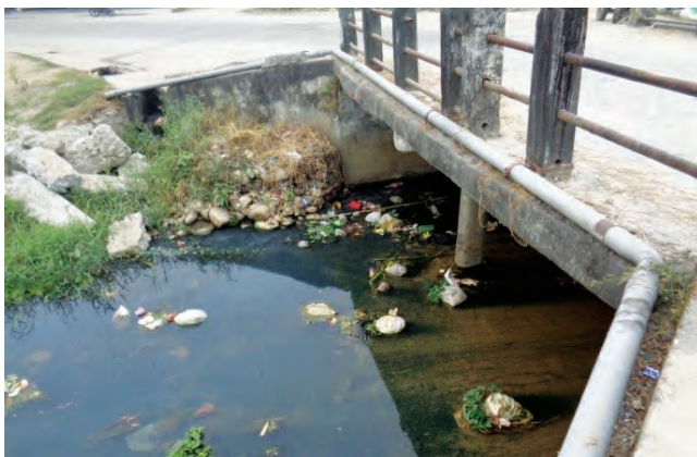
Photo 10. Polluted river due to waste disposal.
