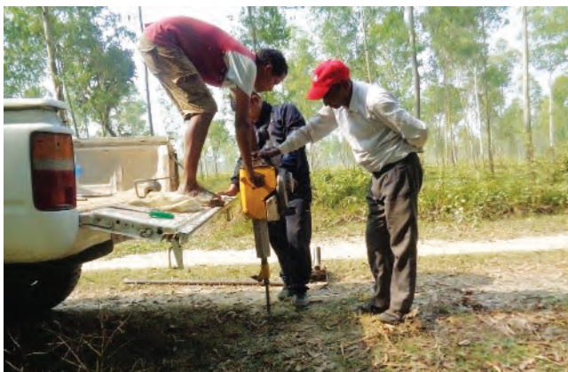
Photo 4. Power auger drilling at the site
