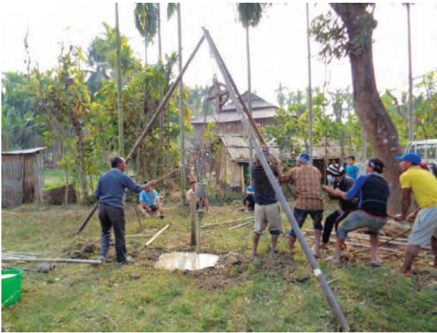
Photo 2: SPT test using monkey hammer
