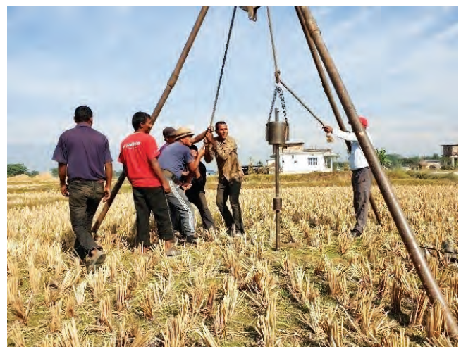
Photo 2. SPT test using monkey hammer
