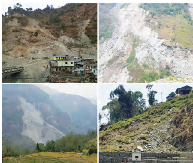
Fig. 2: Landslides observed during fieldwork.
