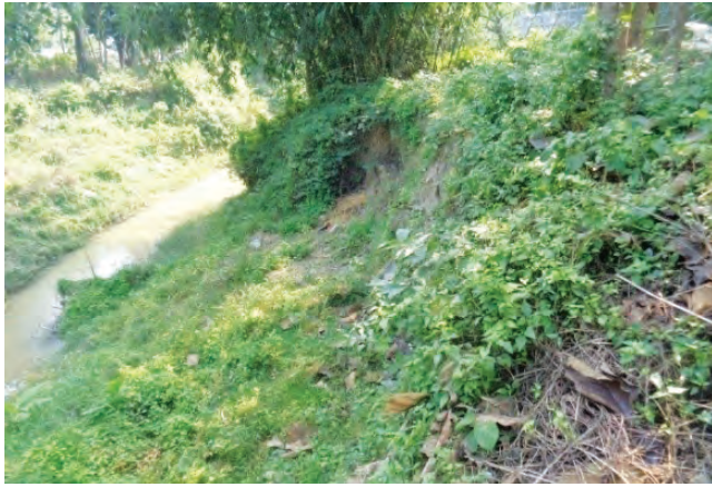
Photo 8. Bank erosion prone area due to small river in Kamal Rural Municipality
